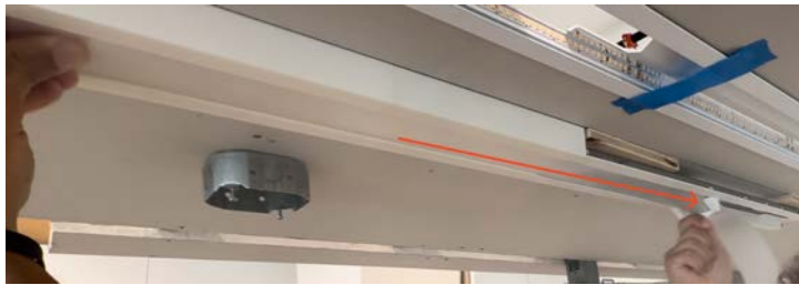
52. Lens is installed
